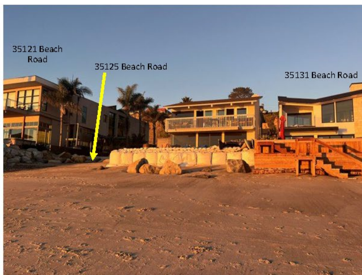
View from beach of subject site and adjacent properties
