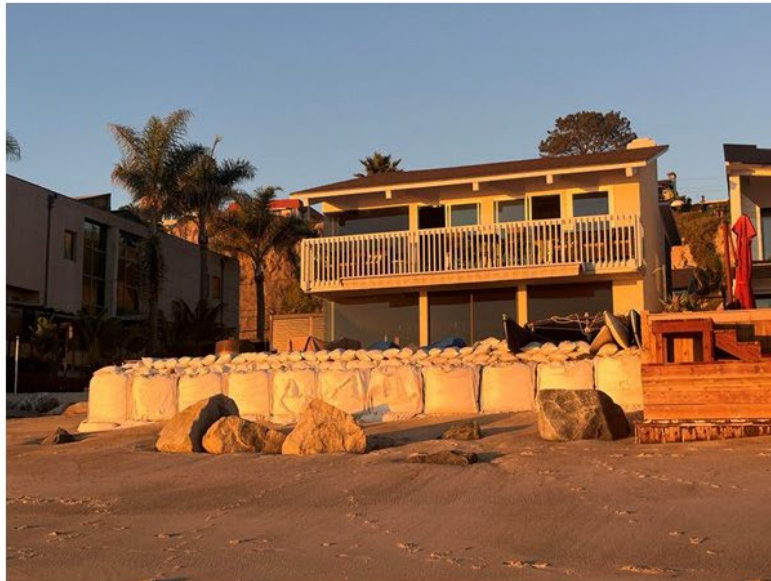
Views north from subject site with existing sand cubes & & rip-rap scour blanket
