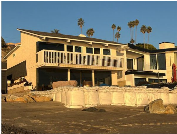
View northeast of subject site with existing emergency CDP sand cubes
