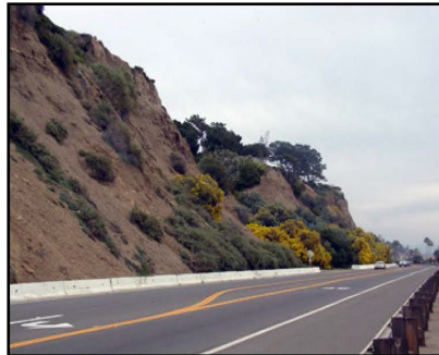
The instability of the Capistrano Bluffs is an ongoing concern. Regulations require development to be adequately set back from bluff edges, and traffic below to be protected from potential landslides.
