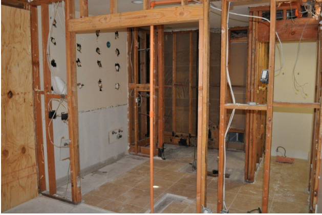
Typical bathroom renovation.
